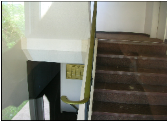
Hallways at front entrance
